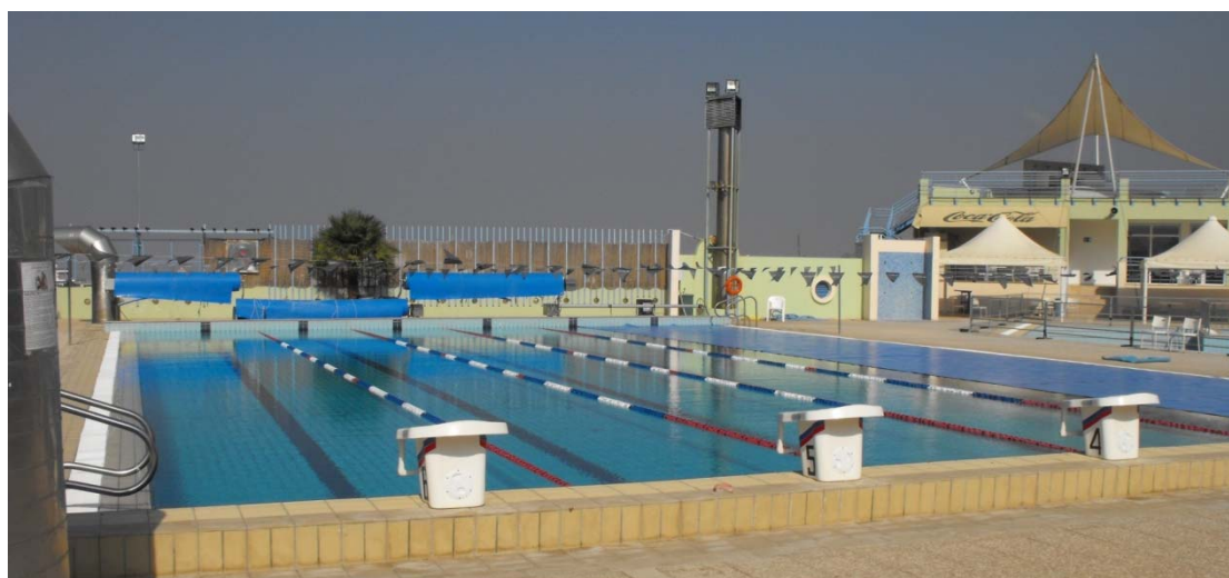
Picture 2. Municipal swimming pool
